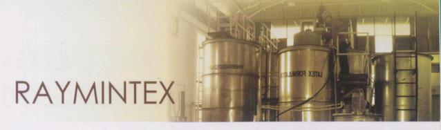
RAYMINTEX plant is a pilot plant dedicated to the prevulcanisation of natural rubber latex by using gamma radiation. The plant was commissioned in March 1996. It is capable of preparing radiation prevulcanised natural rubber latex (RVNRL) up to 6000 tonnes annually, if loaded with 1MCi of radioactive source cobalt-60, to be supplied to natural rubber latex-dipped product industries for the purposes of promotional commercialization and technology transfer.
