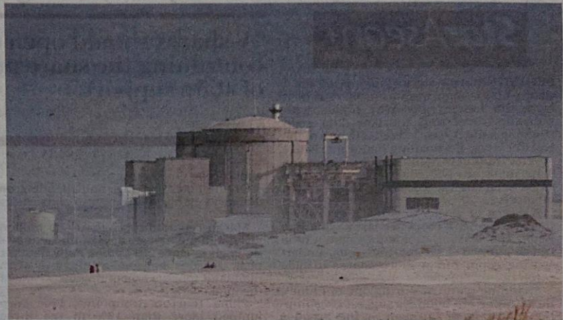
Possible option: A file photo of the Koeberg nuclear power station near Cape Town. South Africa intends to extend the life of the plant by another 20 years. — AFP
